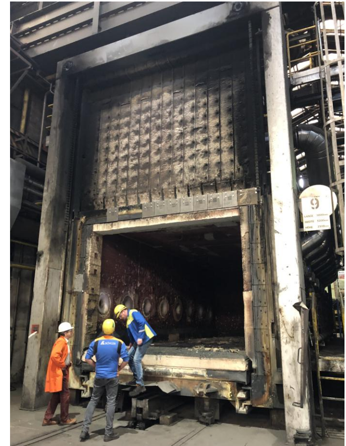
Furnace survey before determining of the final modernization measures
